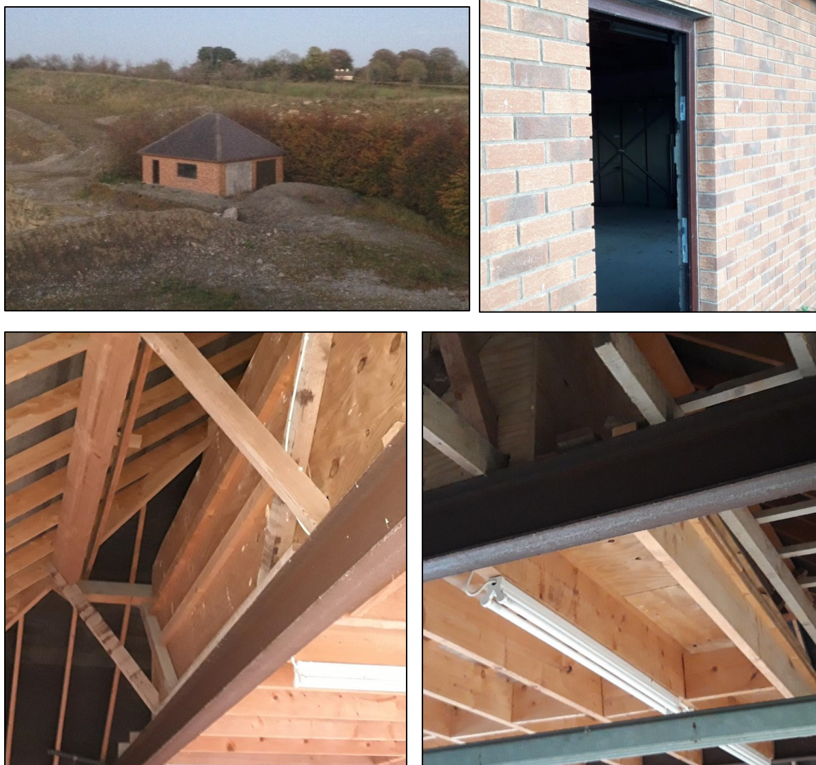
Plate 2. Disused garage showing internal structure of building.
